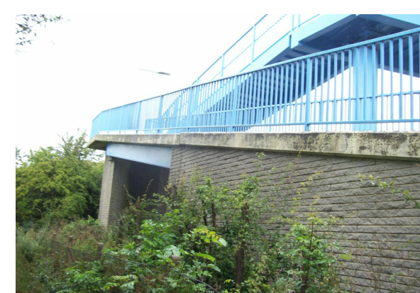
Photograph 8 South elevation of the ramp
