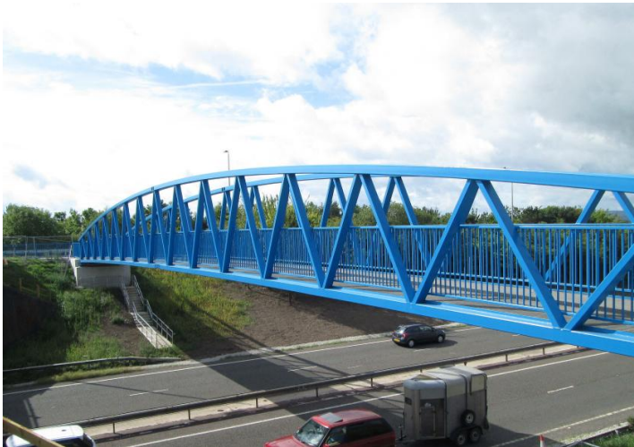
Figure 4.1: Typical Bow Truss Type Footbridge
