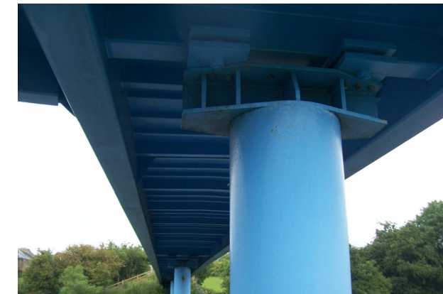
Photograph 6 Bridge Soffit- Connection details between pier and deck
