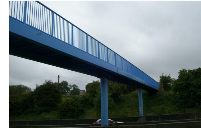
Photograph 9 South elevation of the footbridge
