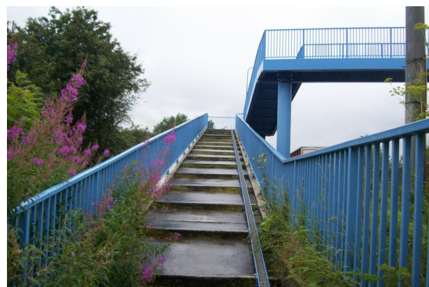
Photograph 7 View of the ramp
